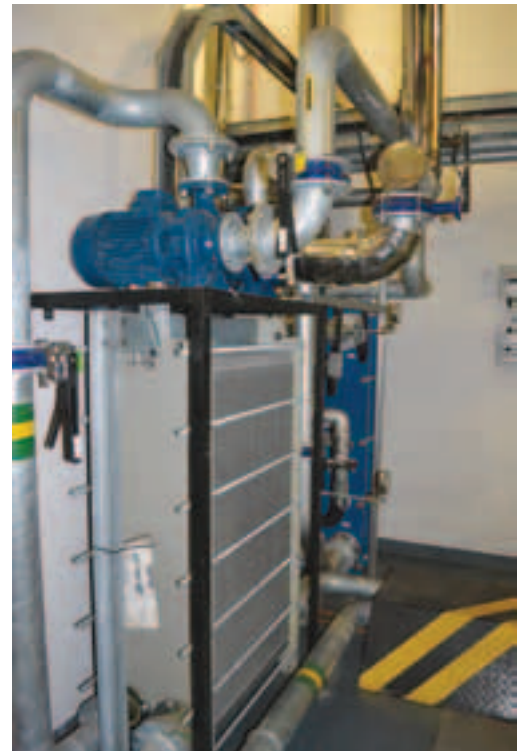
Plate heat exchangers make use of rejected heat from the engines' cooling systems for low temperature domestic hot water. GE Jenbacher gas engine business believes that a 'trigeneration' approach can result in net efficiencies of above 80%.
