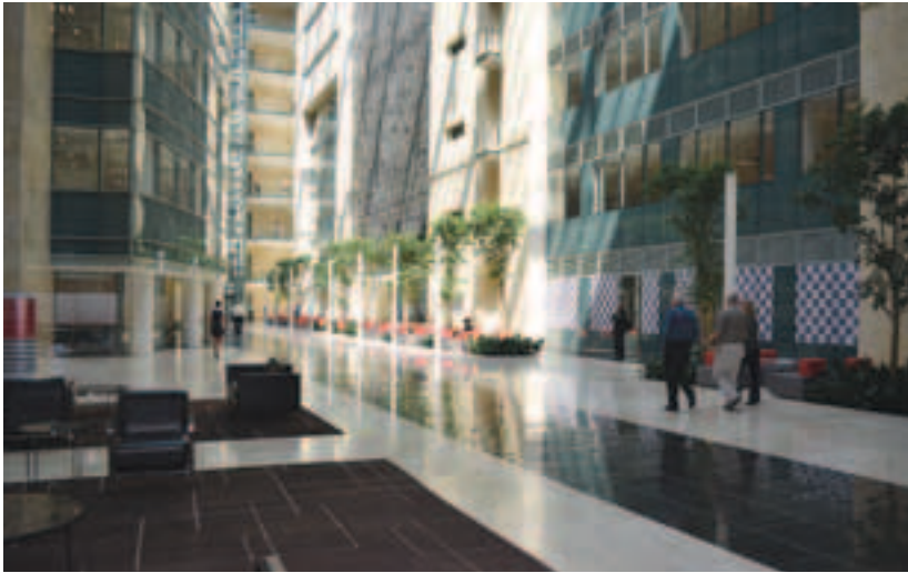
The new Absa Towers West building, one of the most energy-efficient buildings in South Africa. The use of natural light is maximised and supplemented by an automatic system that measures the lux levels and maintains comfortable working light.
